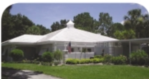
AUGUSTA VILLAS AT THE PLANTATION – The 3BR home has been highly updated w/real wood floors, new carpet & large tile on the diagonal. $199,900 N5769678
